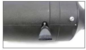
17. Install the duck bill drain onto the brain bracket and secure with the provided tie wrap.
